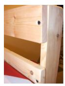
Once you have assembled the ladder it is ready to be fixed to the siderail. Now each floor level is different. Again two holes are there in the side rail ready for fixing.
