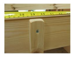
Attach the two guard Rail Supports.
